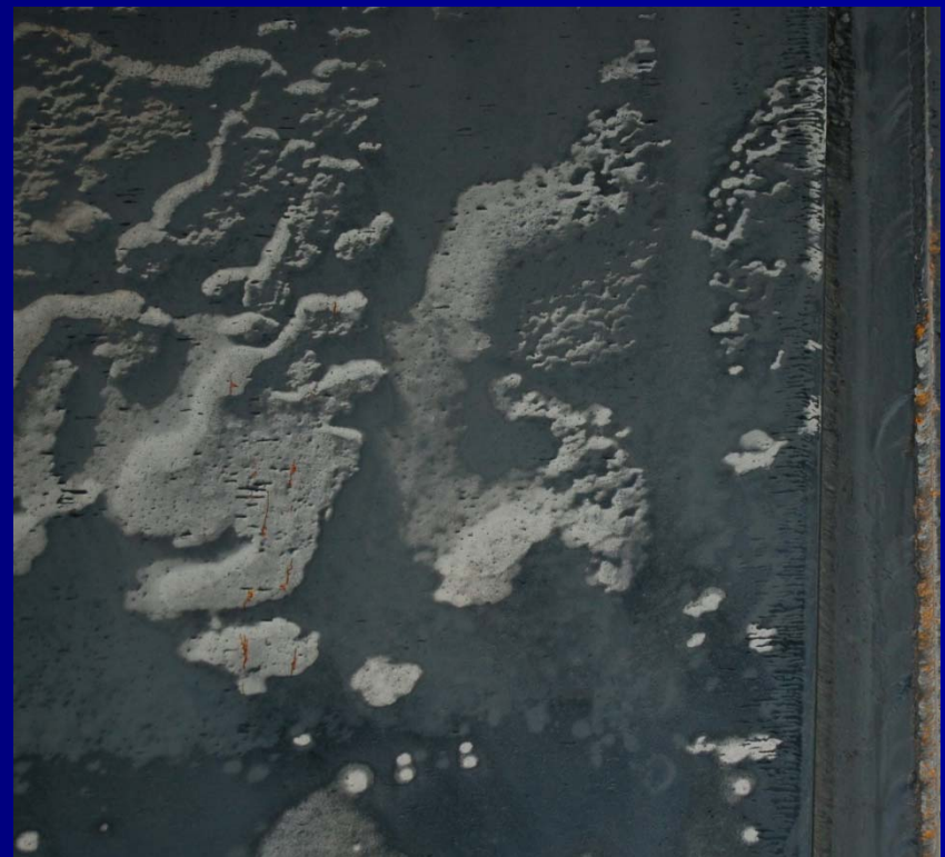
Observed Corrosion in Lenzie ACCs
