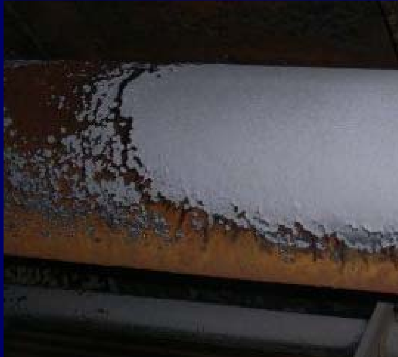
Conventional Condenser Oxygen Corrosion
