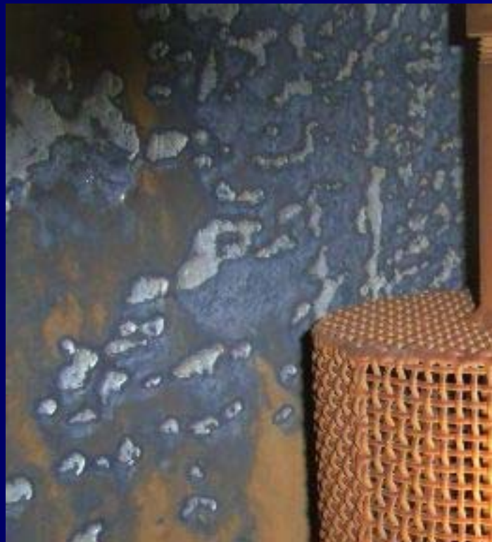
Conventional Condenser Oxygen Corrosion
