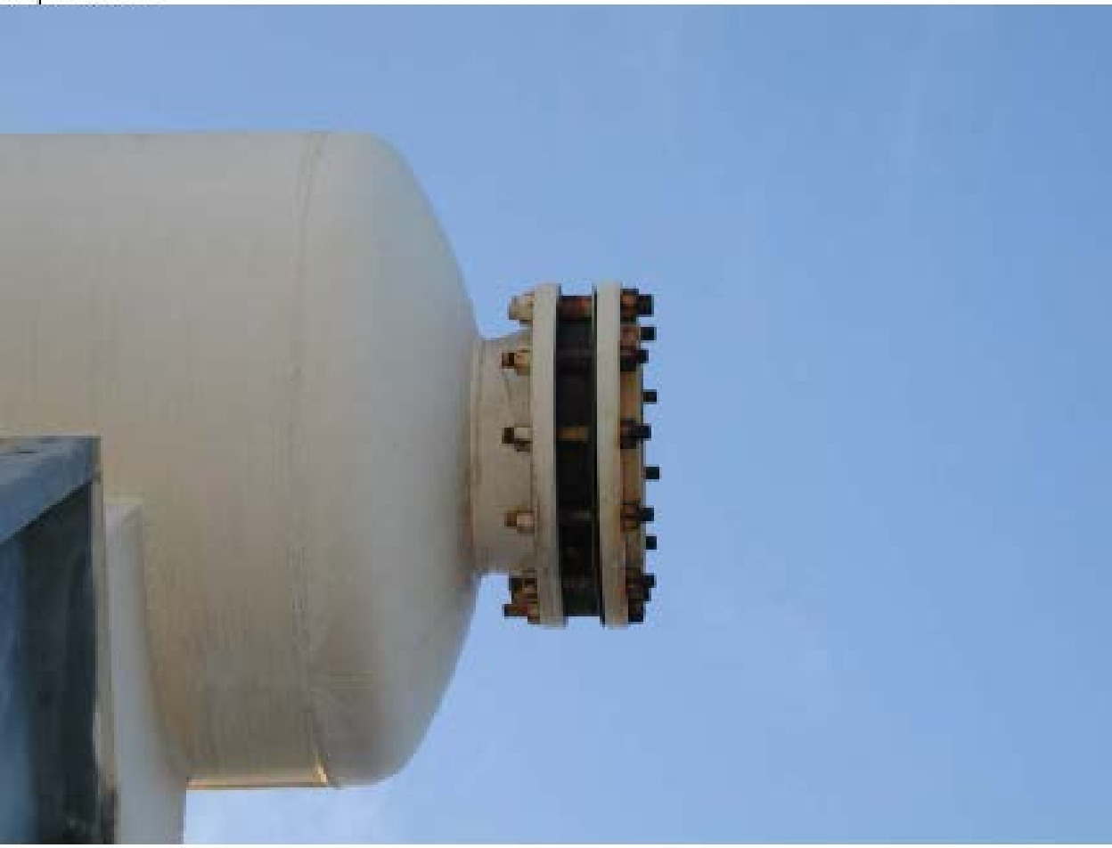
Possible small leak at rupture disc flange, Note the cooler stud and nut (color red)
