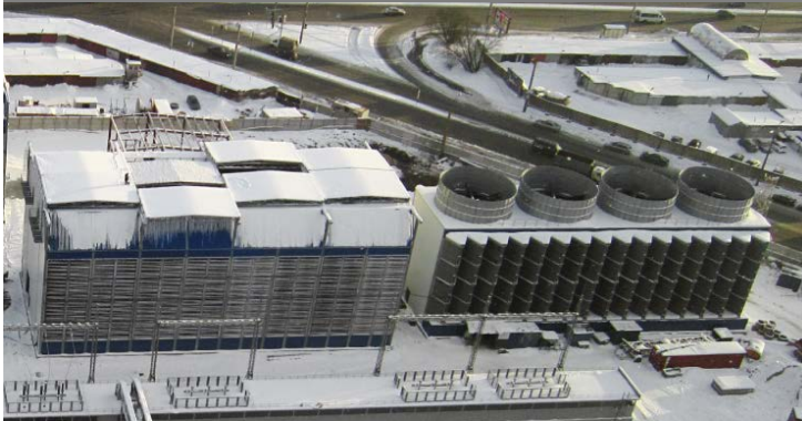
2 × 180 MW e Pervomajsk CHP, Russia freeze proof up to -42°C
