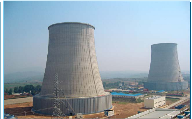
2 × 600 MW e Yangcheng TPP HELLER System with surface condenser
