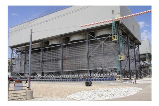
Expected unit performance is 10 MW net increase at 105°F ambient temperature with a 25°F ACC inlet air temperature drop operating 40 hours per year.
