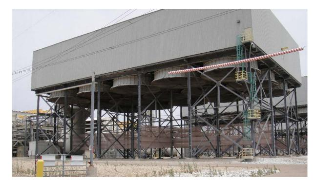
Wind velocity & direction have effected ACC performance during hot ambient conditions. Wind screen placement has improved ACC performance.
