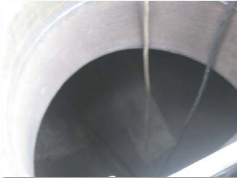
ACC Duct Showing Passivation after SigmaBlow™
