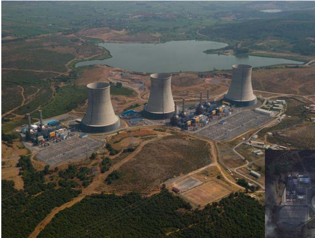
Intergen (Developer) and Bechtel (EPC) 2400 (3x800) MW Gebze & Adapazari CCPP: Largest CCPP with Dry Cooling
