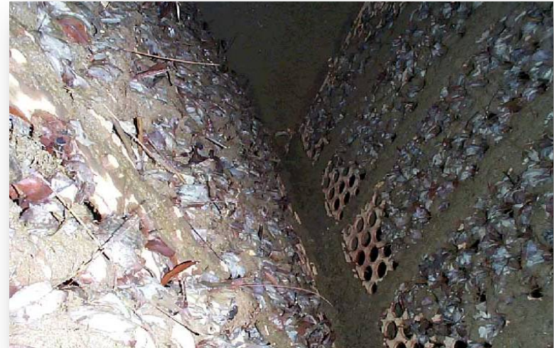
Flow reduction due to macrofouling
