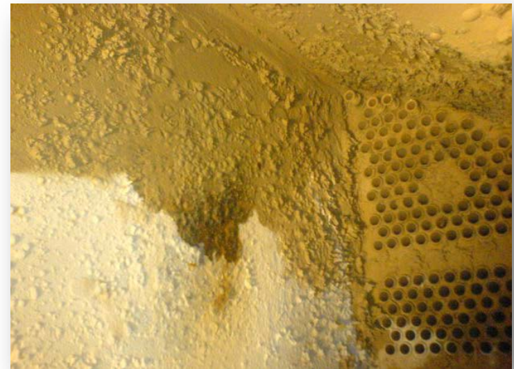
Scaling distributed throughout condenser
