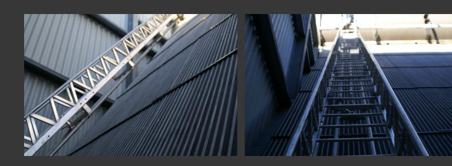
Notice the high pressure spray piping running the length of the ladder.
