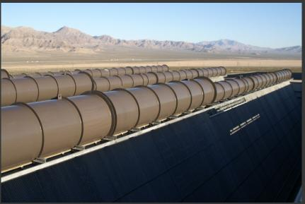
Part of the inspection is rupture disc's and expansion joints (as can be safely reached).
