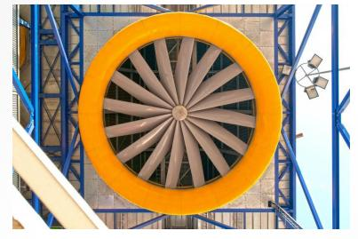
Quote: EON won the "ERNIE" energy efficiency award on Nov 15, 2012. The jury concluded that the overall plant efficiency was worth the ERNIE. This due to a combination of the increased steam flow and the Whizz-wheel® fan providing 20% more air with the same motor power.
