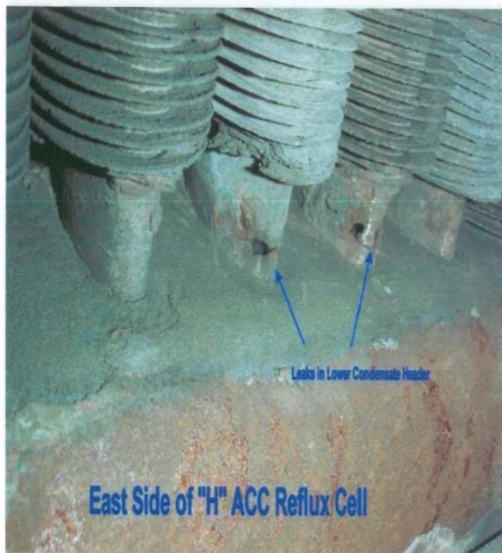
Tube Holes at Tube/Header Connections
