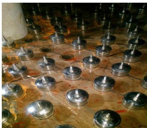
Figure 4. Replacement of strainers (Effluent)
