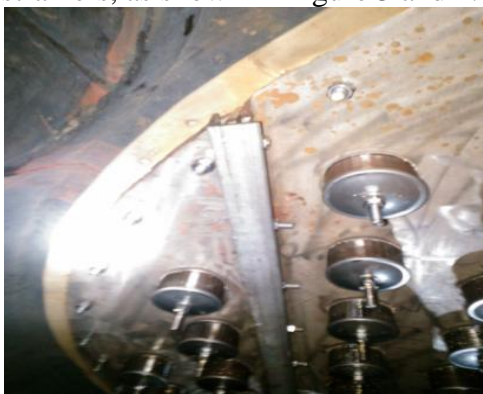
Figure 3. Installation of angle steel at plates gap (Influent)
