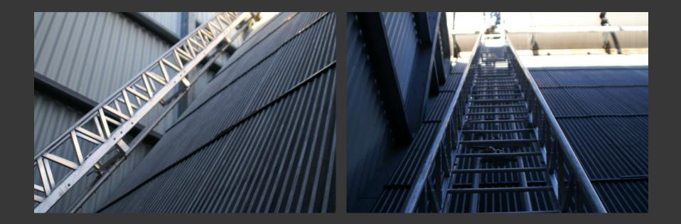
Notice the high pressure spray piping running the length of the ladder. Valves give choice to which section will be cleaned, upper, mid and lower.
