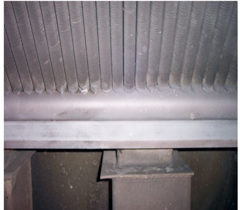
Holes Repaired and Epoxy Painted
