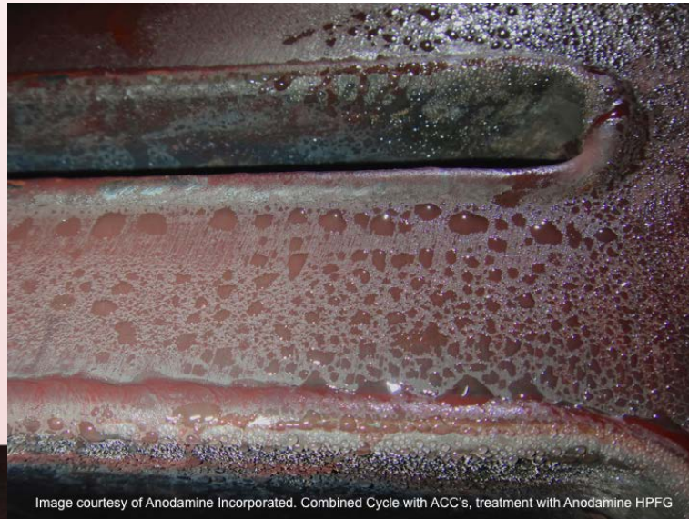
Image courtesy of Anodamine Incorporated. Combined Cycle with ACC's, treatment with Anodamine HPFG
