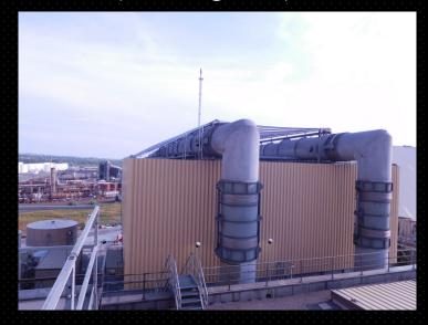
Screen Elevation above Steam Distribution Duct @ ~75 ft (above grade)
