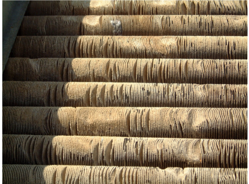
Lime stone by water spraying over bundles Very hard to be removed
