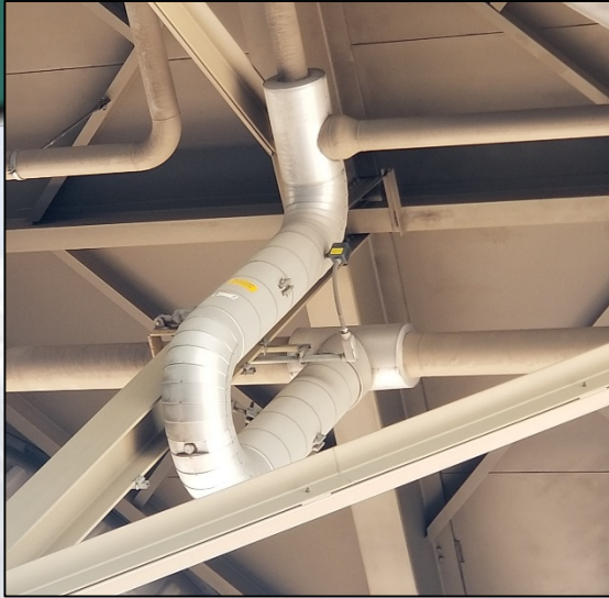
Insulated & heat traced loop seals
