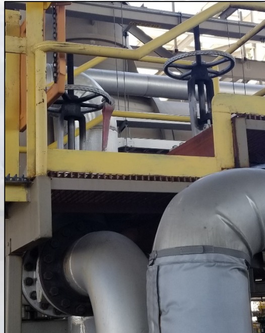
Hogger isolation valves: reduce atmospheric leakage into ACC.
