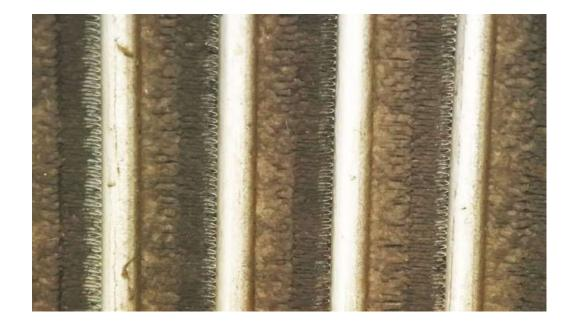
This illustrates the closure of many Air channels of the bundle, result less air for cooling and a higher flow resistance.
