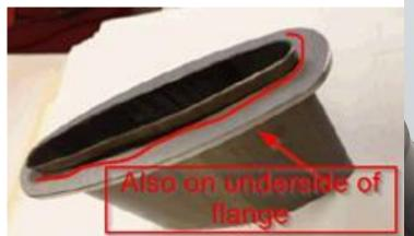
Sleeves Installed by Conco 2017 & Re-installed 2019 (Higher Temp RTV)
