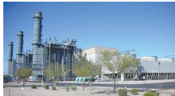
1. New Harquahala Generating Co is an 1100-MW plant with three 1 x 1 combined cycles powered by Siemens Energy SGT6-6000G (W501G) engines
