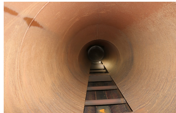
Upper steam distribution duct 5 Feedwater treatment regime: AOT DHACI rating = 1
