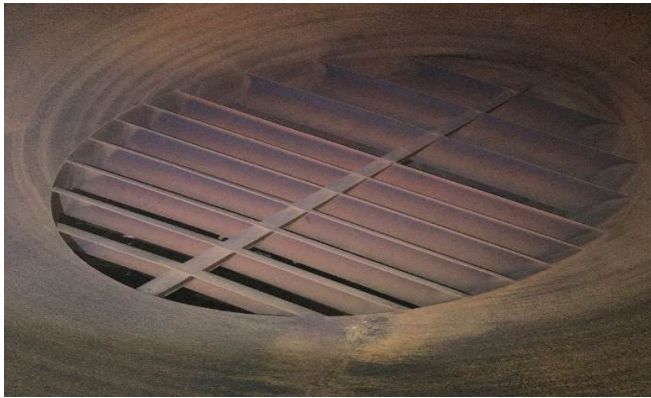
Steam distribution duct 1 inlet louver Feedwater treatment regime: AVT(O) DHACI rating = 1
