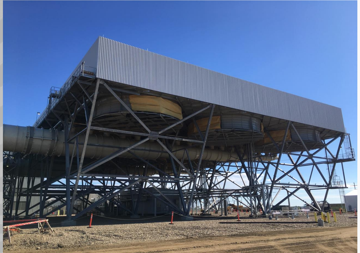
INNOVATIVE STRUCTURE ACC
