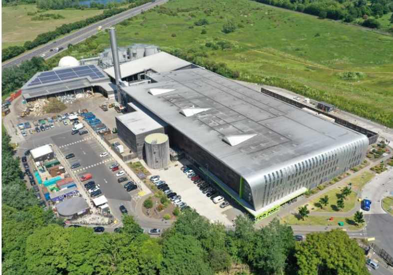
EcoPark Surrey – Gasifier & Anaerobic Digester (AD)
