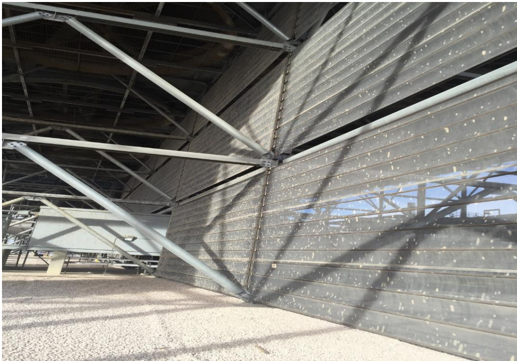
Figure 13: Screen wall installation
