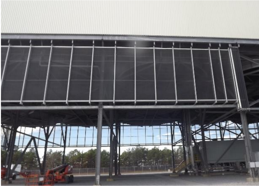
Figure 14: Motorized wind screen designed to reduce fan blade stresses and to allow adjustments as a function of wind speed
