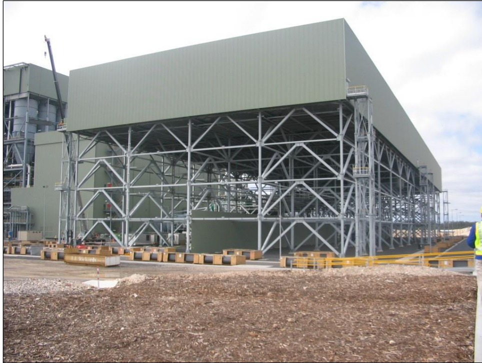
Figure 16: Wind cross at ground level
