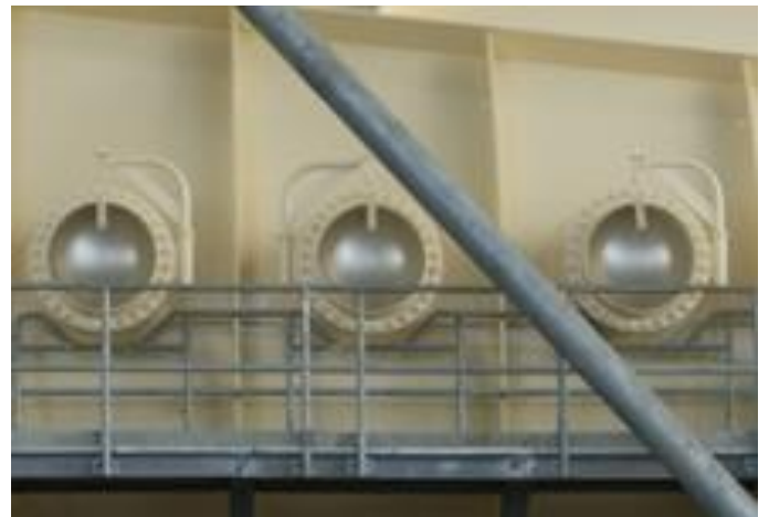
Figure 19: ACC rupture disks
