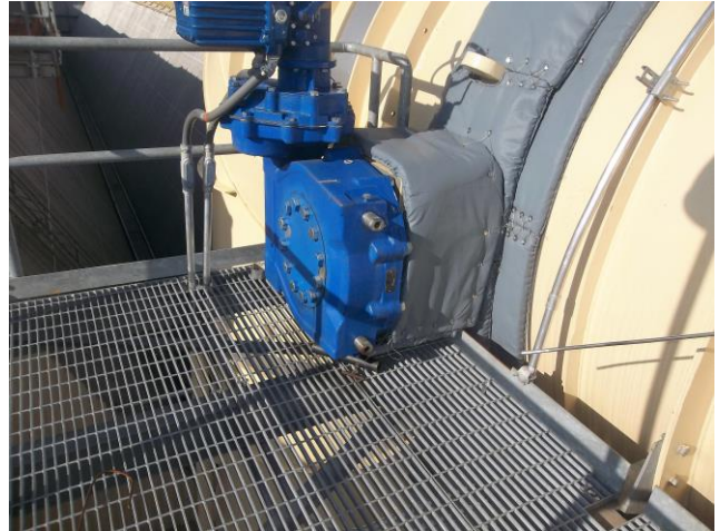
Figure 12: Duct isolation valve
