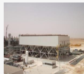
Solar Power Plant In North Africa
