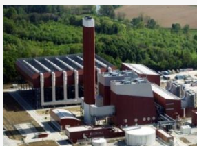
Combined Cycle Power Plant in Europe
