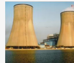
Field Erected Natural Draft Cooling Tower Class 800
