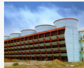
Field Erected Cooling Tower Class 1000 Concrete
