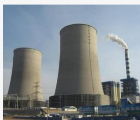
Coal Fired Power Plant – Indirect Dry Cooling – In China
