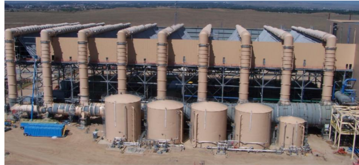
Generic/typical Air Cooled Condenser Design
