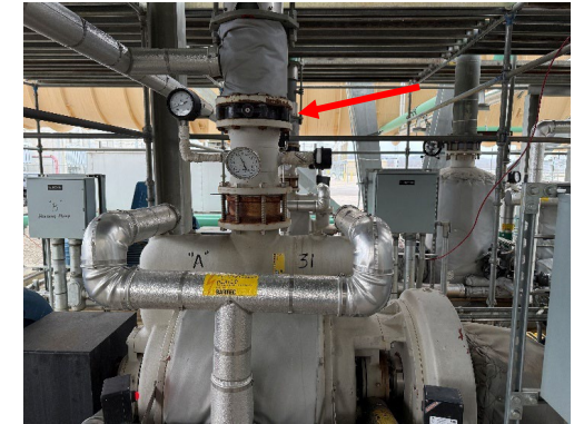
Vacuum Pump Iso Valve
