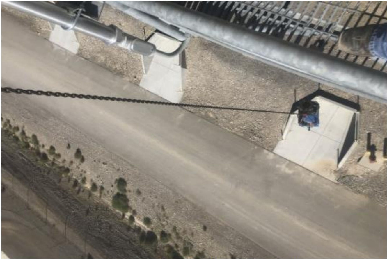
Lowering 2H ACC fan gearbox to the ground
