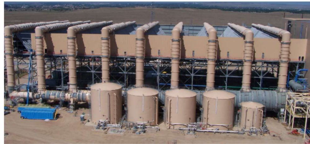
Generic/typical Air Cooled Condenser Design
