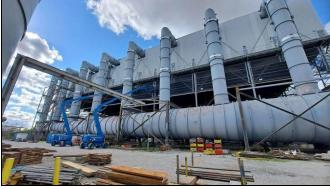
A tour is planned of the ACC at Coryton Station, an 800-MW 2X1 combined cycle gas-fired powerplant with a 40-cell air-cooled condenser, allowing  $\sim$ 95% less water consumption than a typical thermal power plant. Coryton Station is about 30 miles east of London.
