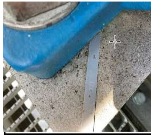
Feeler gauge beneath foot of gearbox
