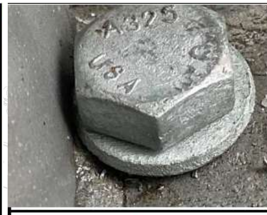
Bolt of baseplate not tightened
